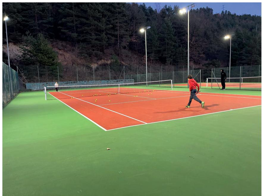
The sports facility in Girona consists of 2 tennis courts, which have been equipped with 12 Cruiser Arena LED luminaires. The aim of the project was to obtain an illuminance of 430Lx and a uniformity of 0.70.
